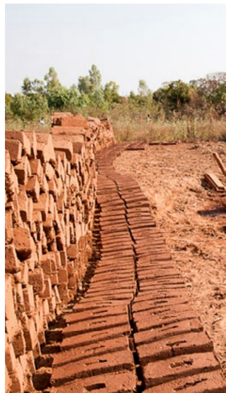
Bricks needed to build a new CBCC in Ng'andu are ready and waiting.
